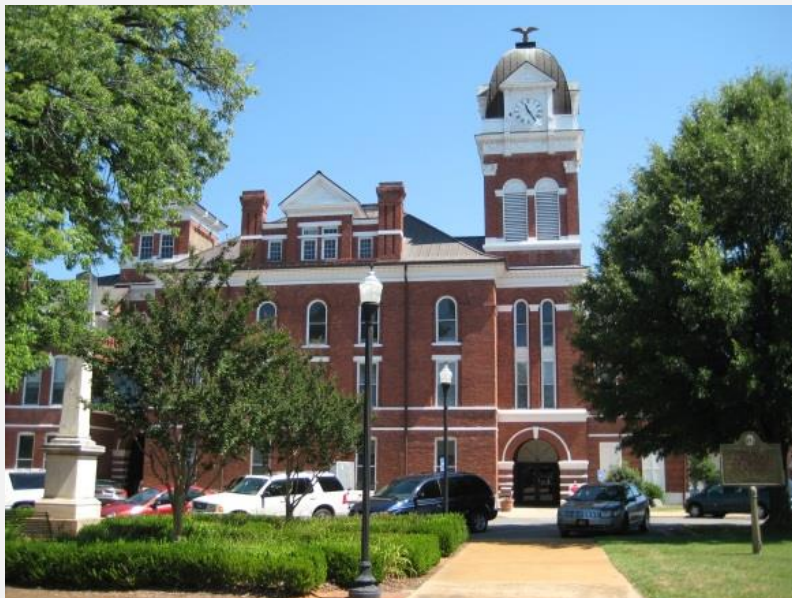
Courthouse restoration projects can improve the appearance of historic landmarks while also ensuring downtowns remain vital.
