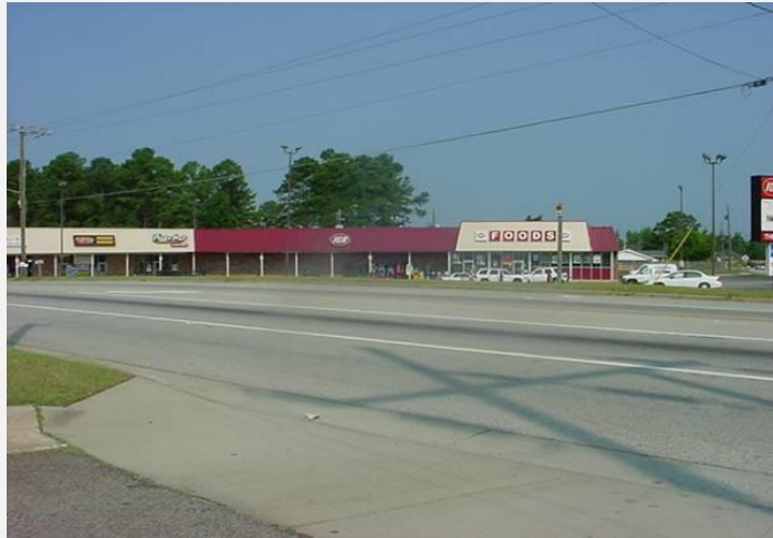
Aging strip commercial centers offer possibilities for infill development.
